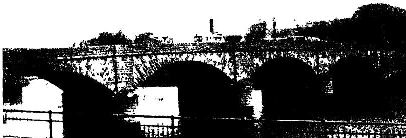
Fig. 6.—The Present Road Bridge at Stirling. A TYPICAL STRUCTURE OF THE PRE-1914 PERIOD.
